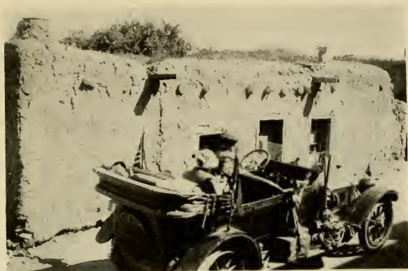
In front of "the oldest house" in the United States, located on a narrow street in Santa Fe, New Mexico, and said to date from 1530. It is of adobe construction—mud and straw—and was formerly two stories in height. A Mexican family makes it its home
